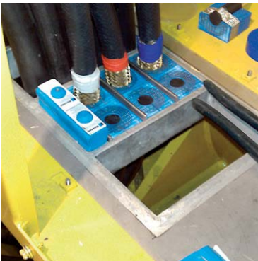
Bonding and grounding: Roxtec BG™ provides solutions for termination of conduits, armored and metal clad cables in control cabinets and junction boxes.
