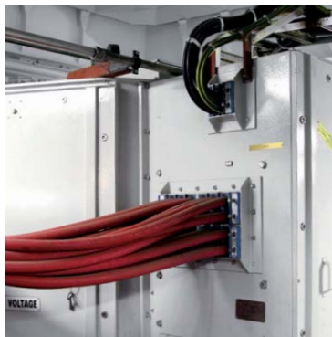
Generators and propulsion system: Roxtec seals are adaptable to fit cables and pipes of different sizes.
