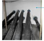
**Beneath floor:** Single power cables sealed air-tight with Roxtec round seals.
