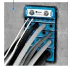
No air leakage in wall beneath floor: A Roxtec G frame can handle a combination of cables for transmission and control.
