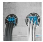
**Foundation:** sealing of power and control system cables going through core-drilled holes.
