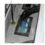
**Raised floor:** sealing of fiber optic and cat 5-cat 7 transmission cables.
